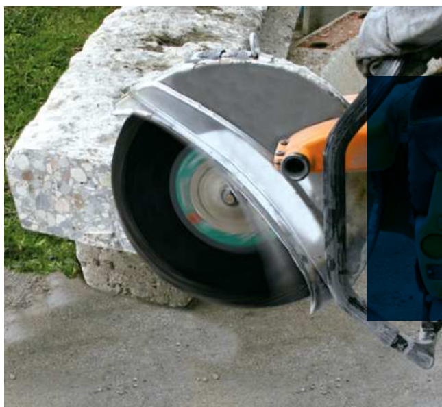
Metalynx PRO Stone wheel cutting a curb.
